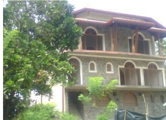
An illegal construction in
